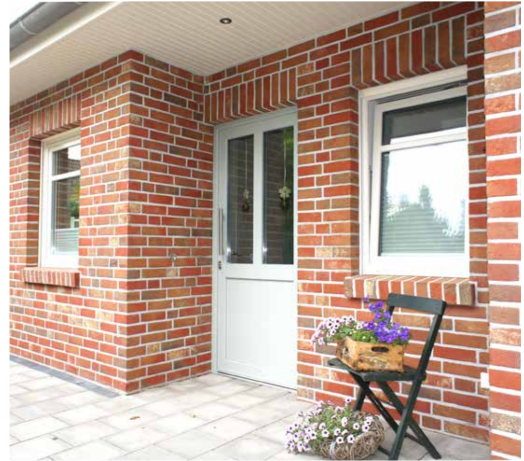
Original Hand-moulded bricks
