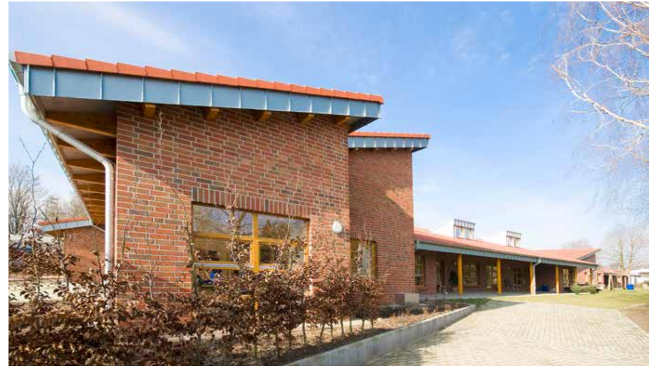
Original extruded bricks
